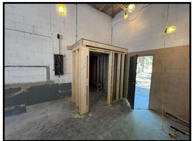
ADA Bathroom Framed
